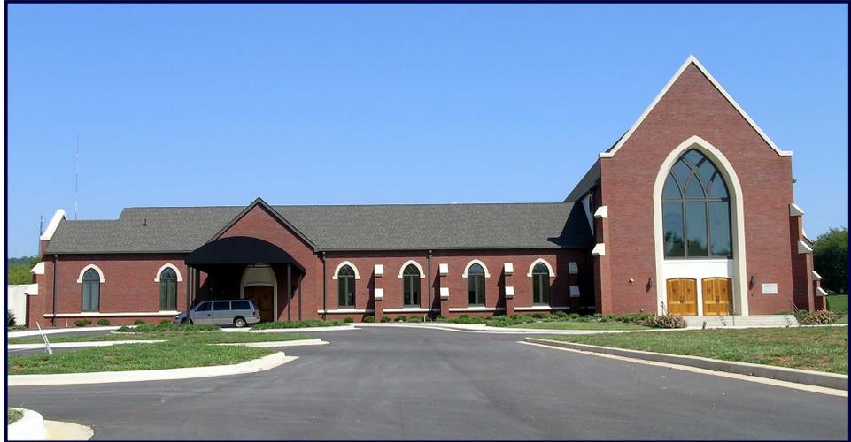
The 3500 square foot classroom wing is concrete block with cast stone and brick veneer, wood truss and shingle roof.
